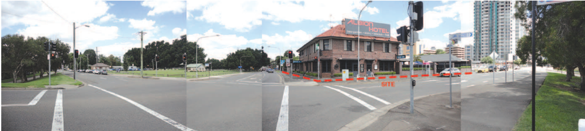
5/ Overall view from George Street
